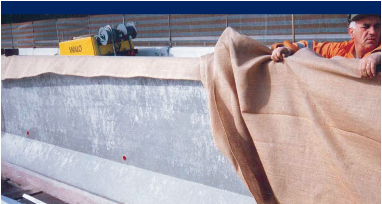
Figure 1. The finished parapet - Ready to use without any kind of after treatment.
