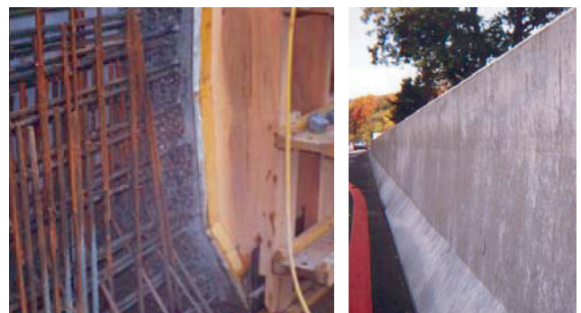
Figure 3. Casting of parapet and finished result.
